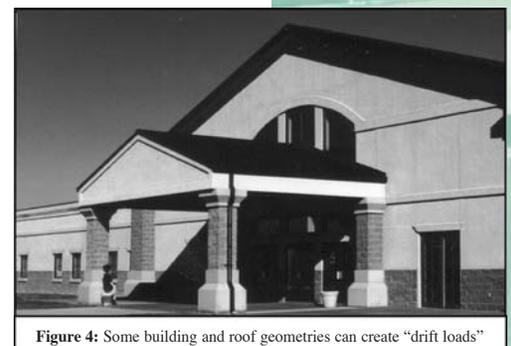
loads to the lower roof. Determination must also be made with respect to using uniform or non-uniform loads in design. Governing building codes should be consulted and appropriate engineering standards and calculations are vital to determine the actual in-service roof loads in all such cases.<sup>1</sup>
